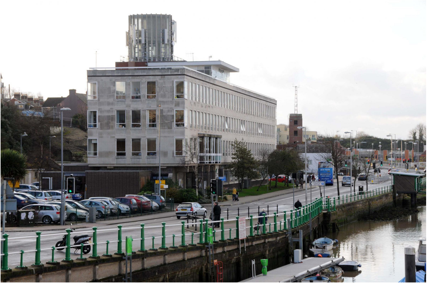
Figure 1 / Existing office building North Quay, Weymouth
